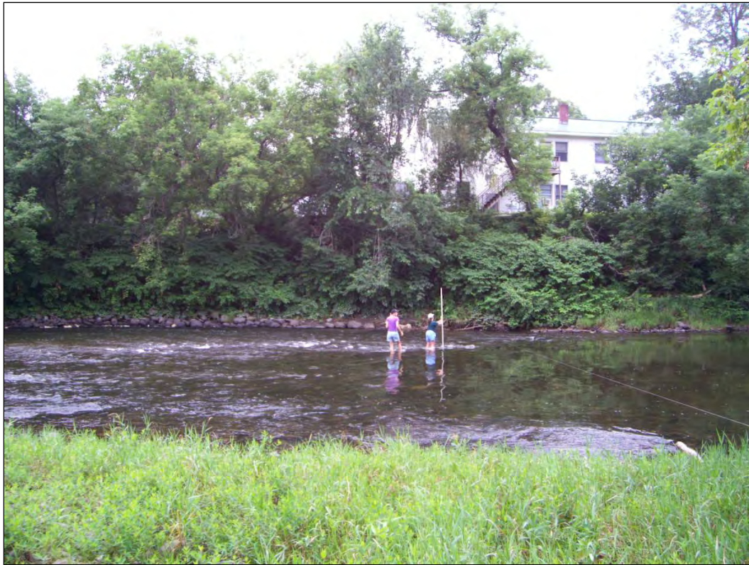
Figure 24. R14-A flows through Johnson Village. Historic channel straightening and floodplain encroachment have resulted in loss of floodplain access.
